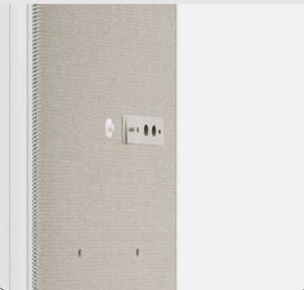
7. Install electrical appliances and sound absorbing cotton
